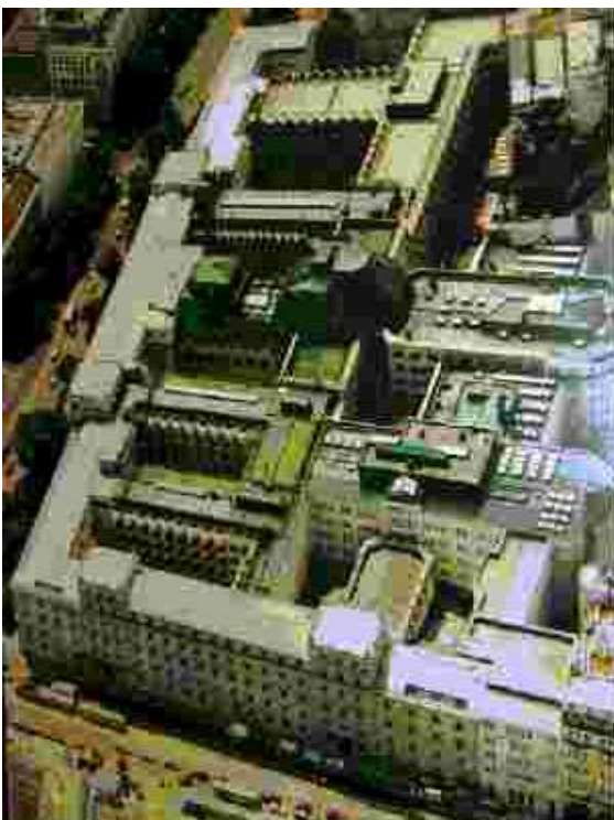
Figure 1: Austrian Federal Detention Centre in Josefstadt, central Vienna- aerial view.
